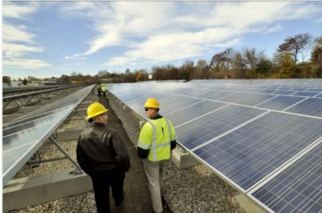
1.8 Megawatt Plant in Pittsfield, MA Largest Solar Installation in New England
